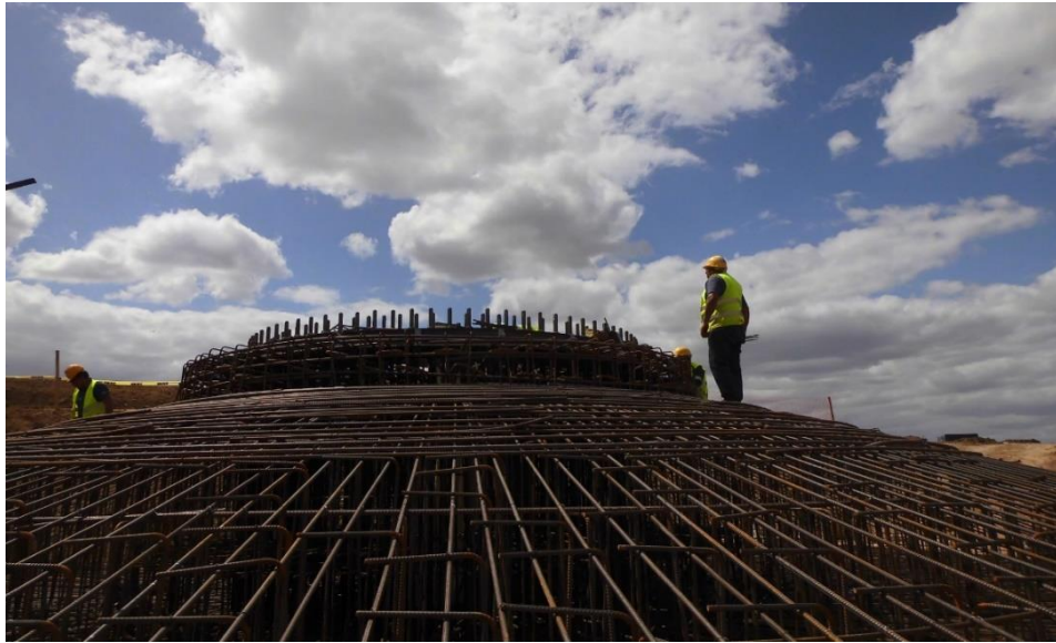
+1000 WIND FOUNDATIONS PER YEAR
