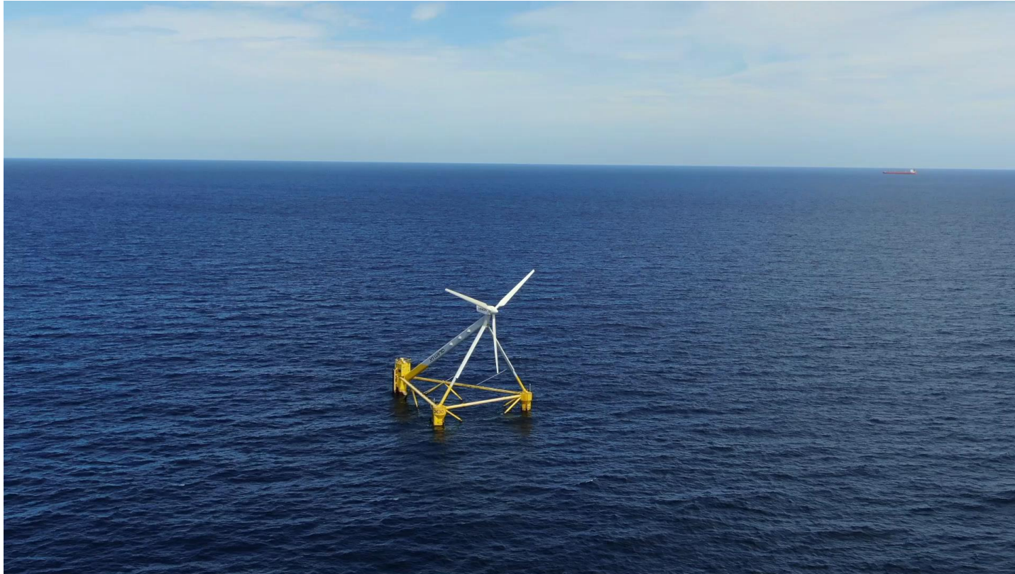
The first fully operational TLP wind turbine platform
