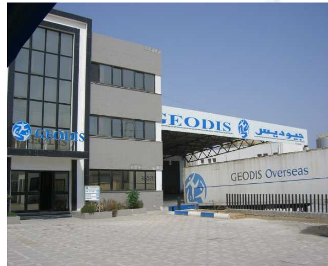
Geodis Tunisia bonded warehouse in Rades
