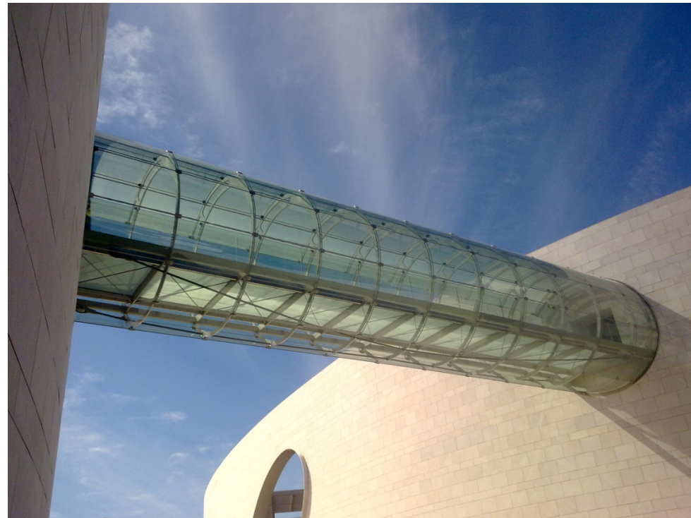
Architectural Steel and Glass
